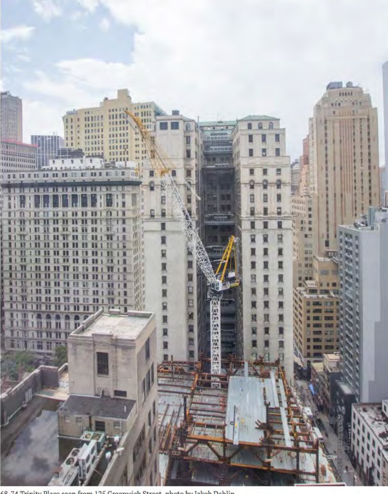
68-74 Trinity Place seen from 125 Greenwich Street, photo by Jakob Dahlin
