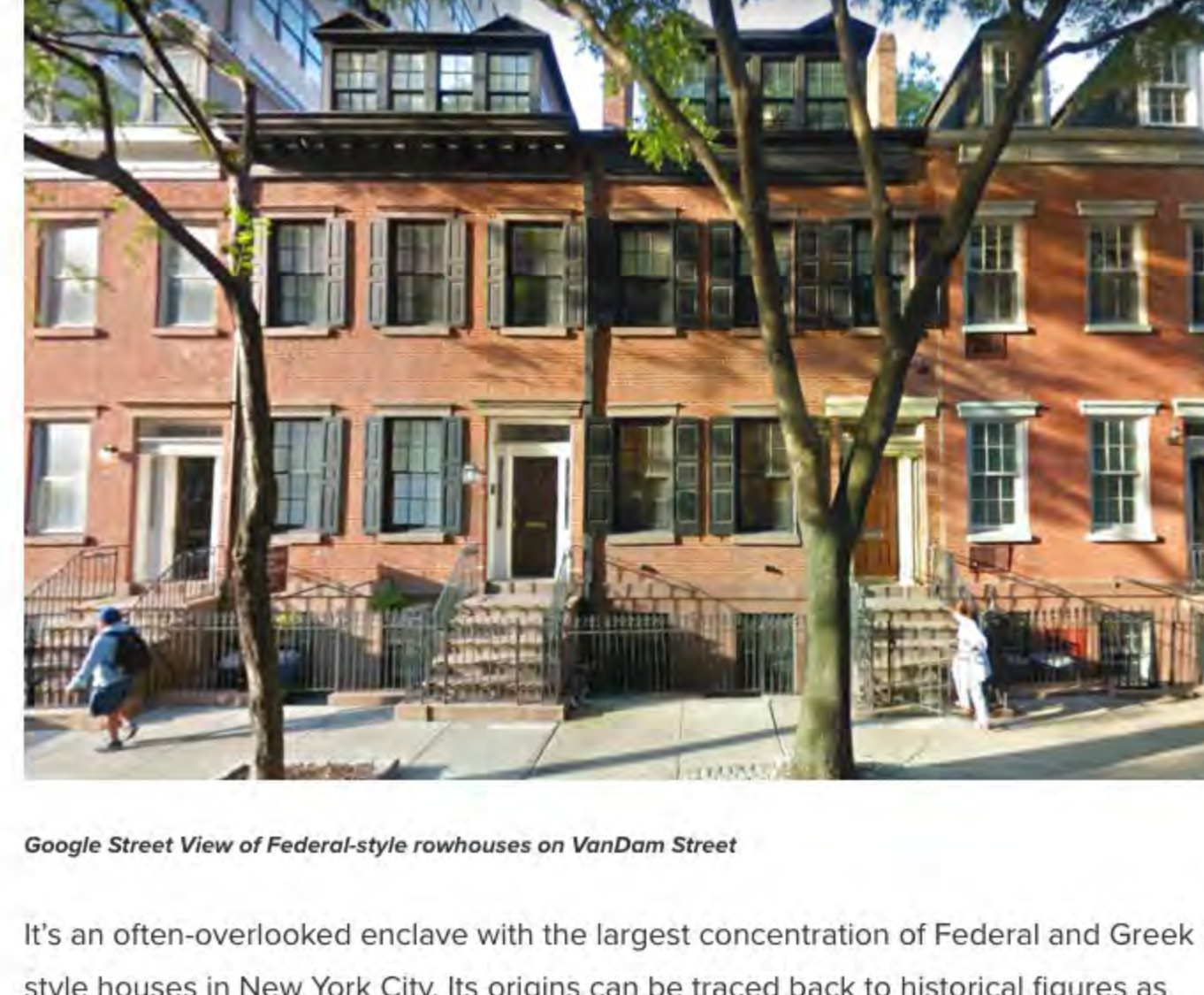
Google Street View of Federal-style rowhouses on VanDam Street
